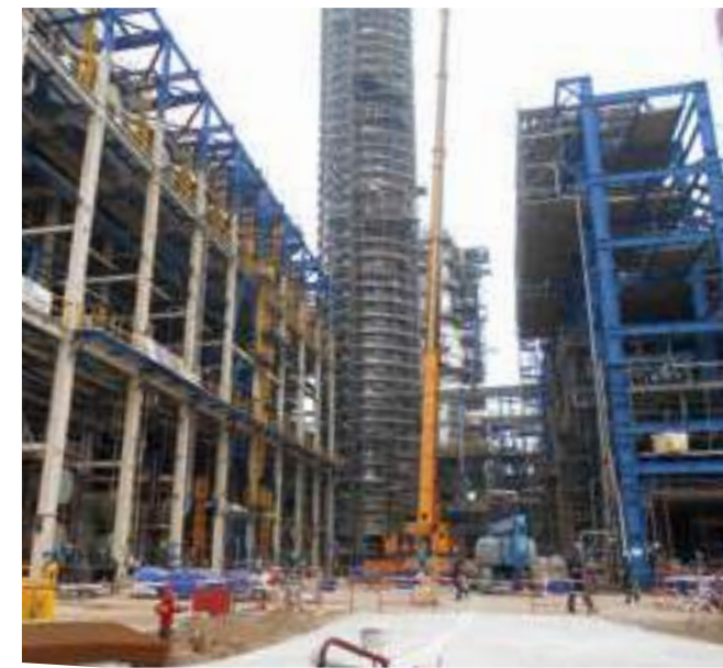
Star Oil Refinery Gemsan - Tekfen - İOT - Vito - Günkön - İlk Construction İzmir, Turkey
